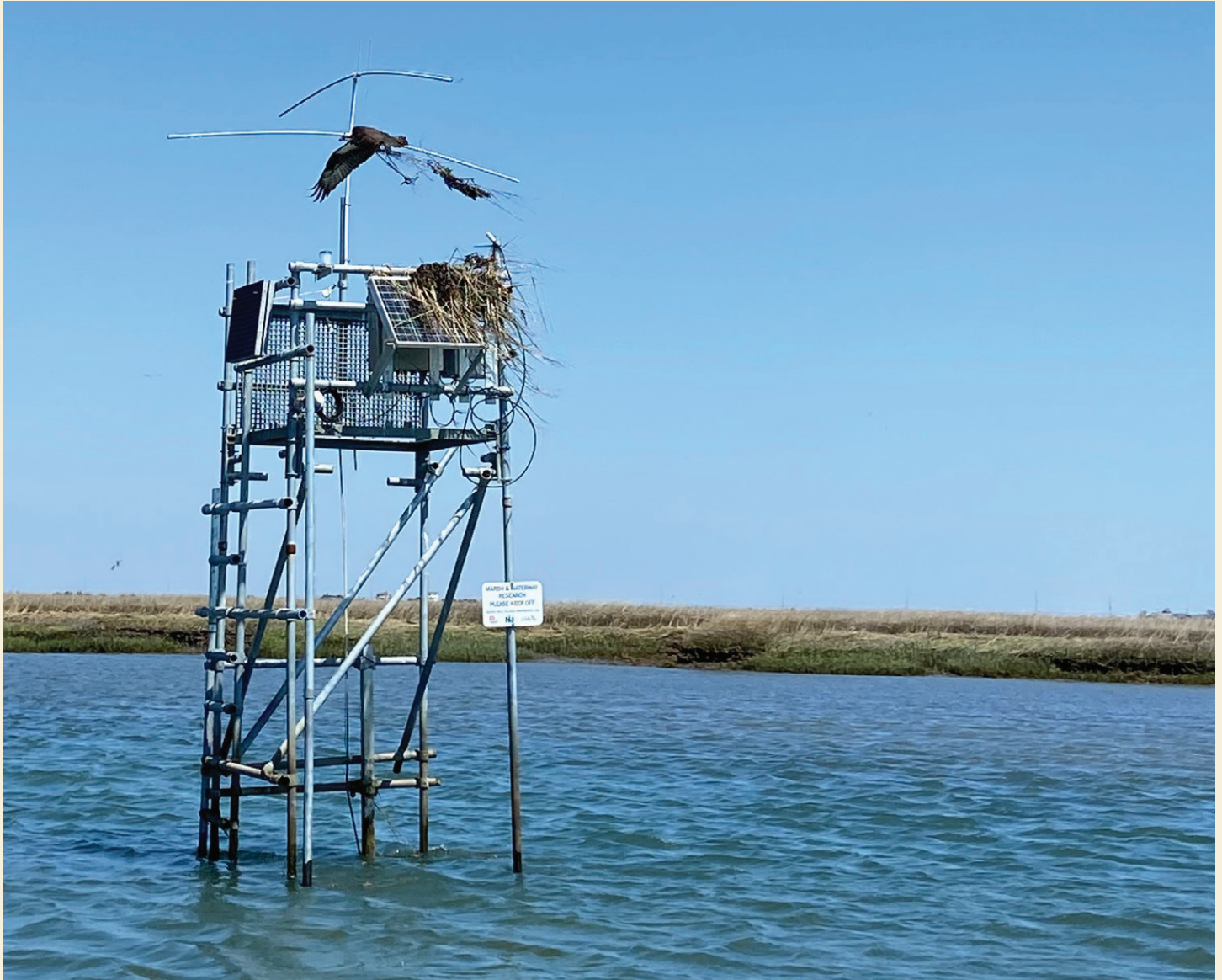
An observational platform installed in a salt marsh estuary in coastal New Jersey (Seven Mile Island Innovation Laboratory). The platform was equipped with underwater sensors that continuously monitored dissolved oxygen, temperature, and pH. Data collected autonomously over a three-year period was used to track how the marsh "breathes" as plants produce oxygen and marsh life consumes it Photo: Jake Supino
